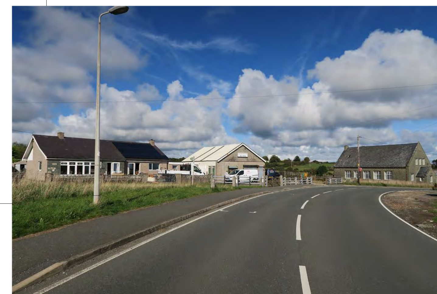
Existing Site Photo 1
